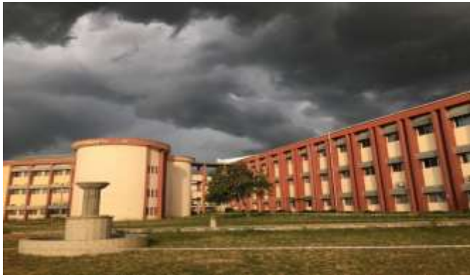
Figure 1: Building Form, Faculty of Architecture University of Jos
