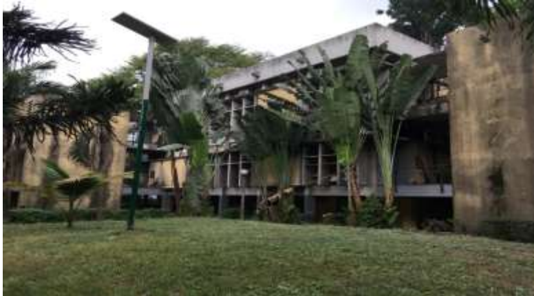
Figure 3: Building Form, Faculty of Architecture, University of Lagos
